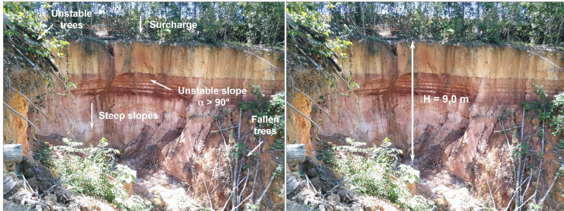
Figure 3. Geometric and geotechnical characteristics of the gully before intervention.
