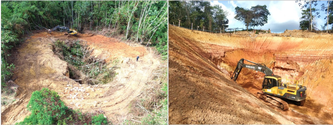
Figure 7. Earthworks (12/08/2023) and slope reshaping (09/01/2024).
